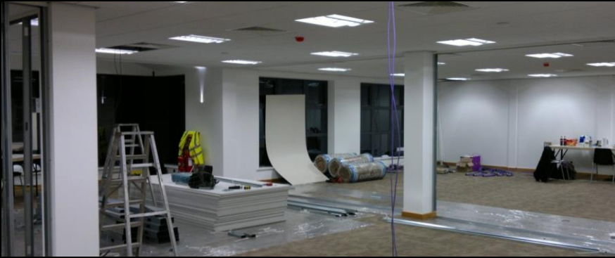
New Space Cabling
